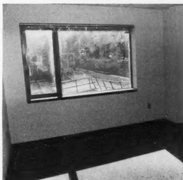
Openable windows for the classrooms.
